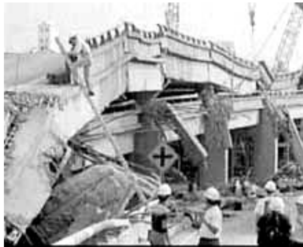
Figure 5. Cypress Structure, Oakland. Damage from the 1989 Loma Prieta Earthquake.
