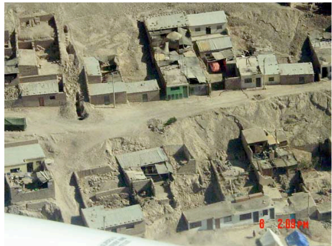
Figure 3. Adobe buildings in Peru were severely damaged in intensity VII shaking in 2001.
