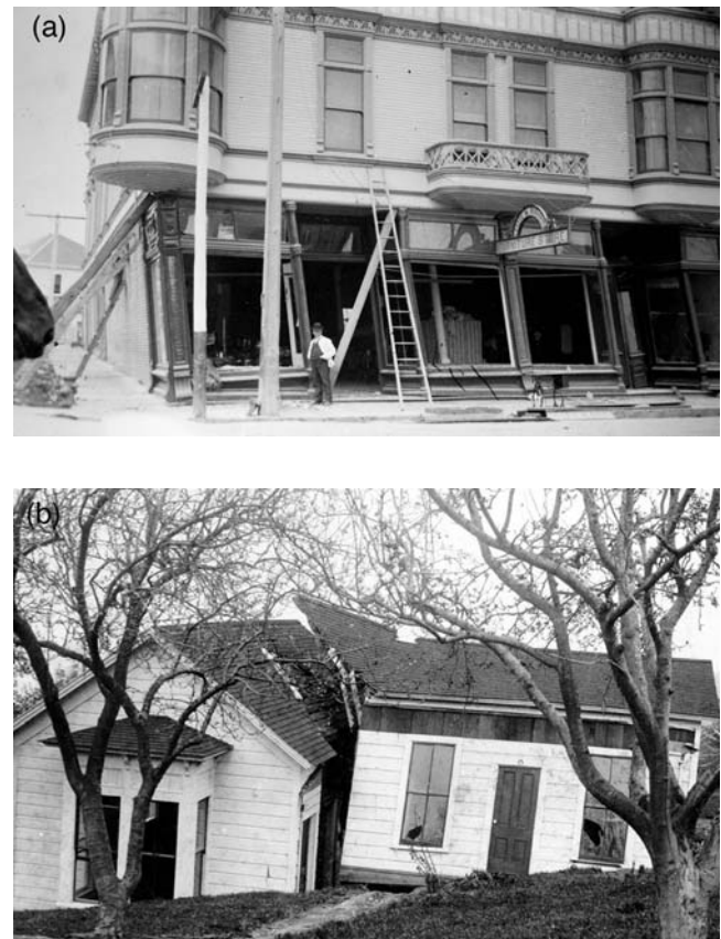
Figure 5. Damage to wood-frame buildings in Ferndale. (a) The Knights of Pythias Hall, repaired after the earthquake, was eventually replaced by a gas station. (b) Unidentified home. Photos by E. Garrett, courtesy Peter Palmquist.
