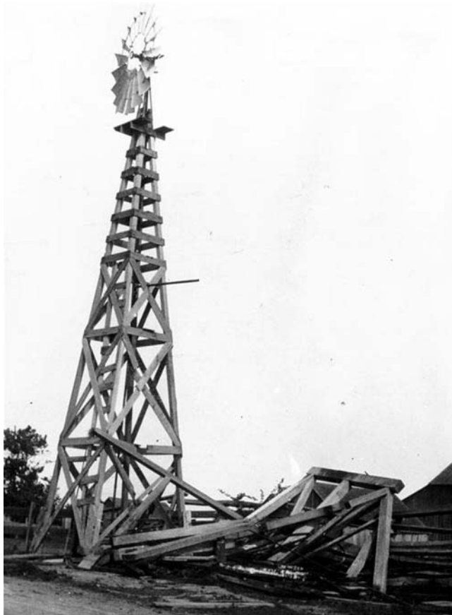
Figure 6. Twin windmills in the Eel River Valley; mill on the right has collapsed. Photo by E. Garrett, courtesy Peter Palmquist.
