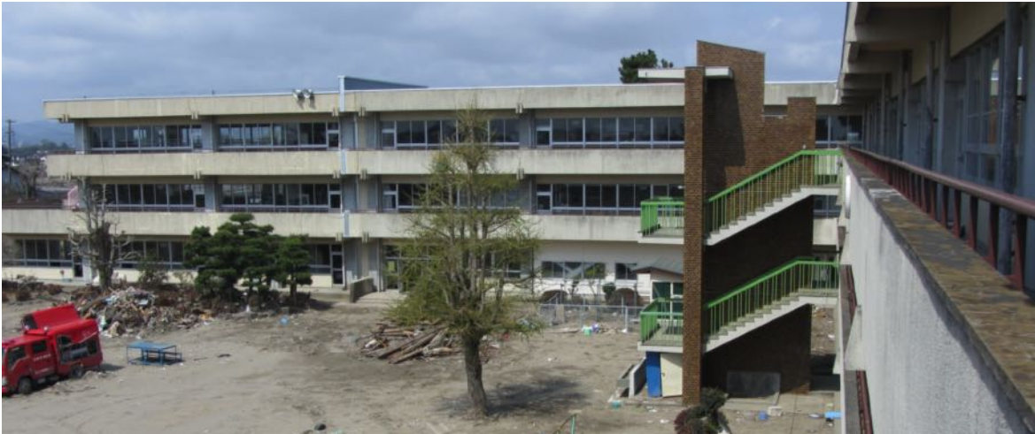
Elementary school at Yuriage. Note exterior stairways that provided the community with access to upper floors.
