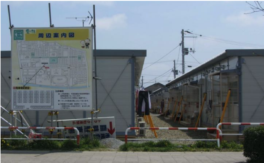
Completed temporary housing, Iwanuma
