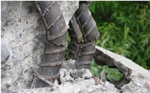
Failed rebar in bridge support near Kaikoura, New Zealand 2017. Repeated loading - unloading cycles during the 2016 M7.8 earthquake contributed to the failure. Photo from EERI Learning from Earthquakes.
